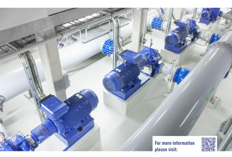
between 14 and 25 per cent. A drive adjusts a motor's speed to precisely match the task's requirements, increasing efficiency.
